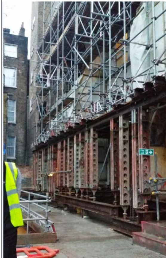
Rear Elevation (under construction)
